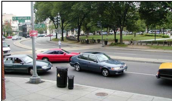
A roundabout is not : 2. A Washington DC style circle, with traffic signal controls
