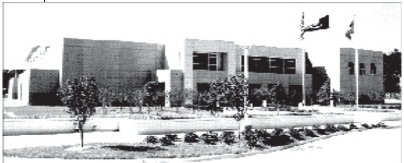
Advanced Traffic Management and Emergency Operations Center 3773 Harding Boulevard, Baton Rouge
