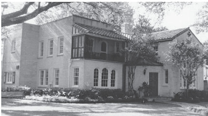
Above: This residential building is located in the Drehr Place National Register District. Drehr Place is significant in community planning and development.
